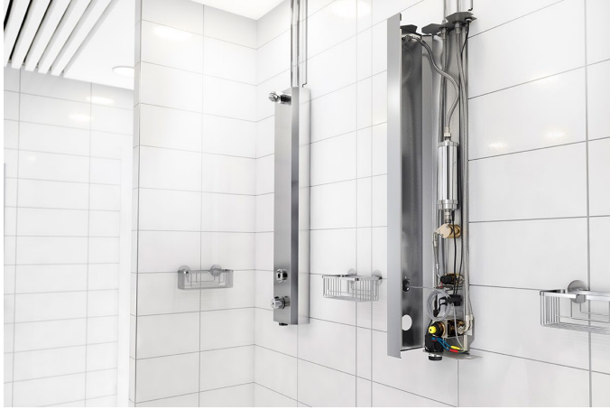
Figure 1.3 - Shower Application - Watersprint purifier installed to add an additional hygienic barrier to protect against plumbing pathogens (e.g., Legionella ) at the point of dispense in a shower. One infection pathway for Legionella is the inhalation of aerosols during showering.
